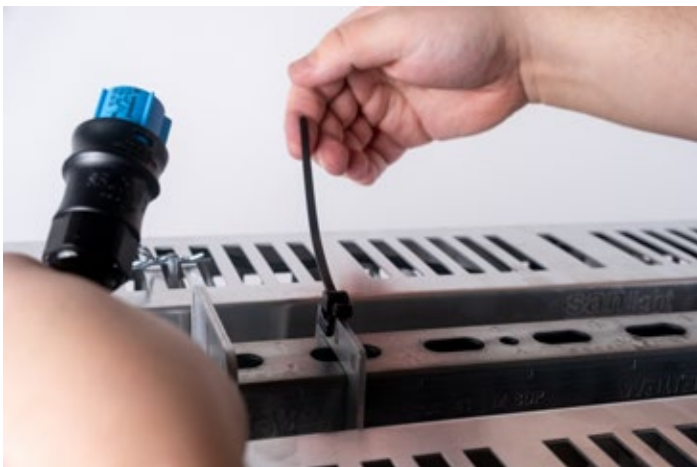
Step 12: Attach the enclosed cable ties to the suspension brackets. Take the dimming cable (blue plug) and attach it.
