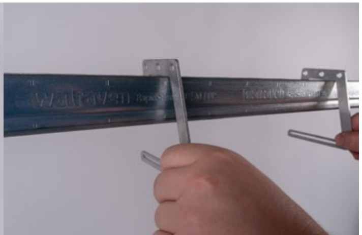
Step 2: Place the driver hanging brackets on the support beam.
