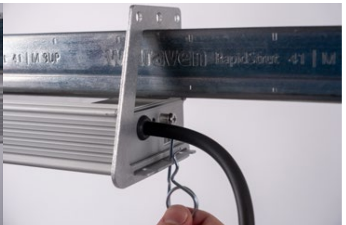
Step 5: Secure front and back end of the driver with the splints in the slot of the hanging brackets.
