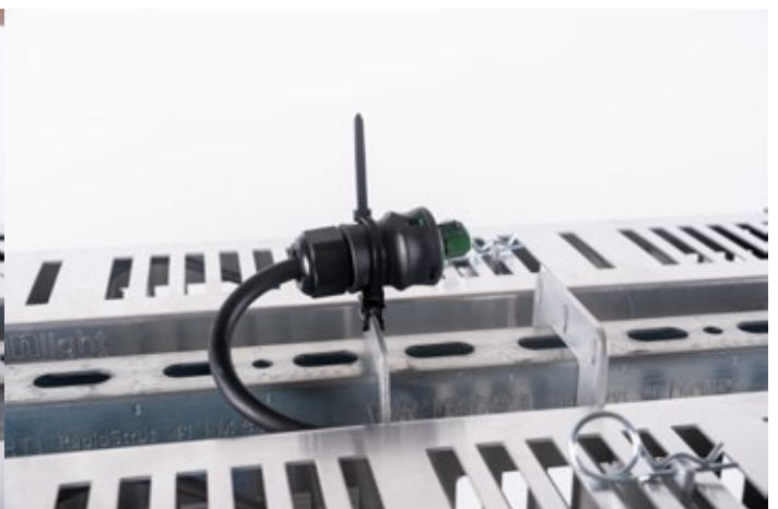
Step 12: Attach the enclosed cable ties to the suspension brackets. Take the AC cable (green plug) and attach it.
