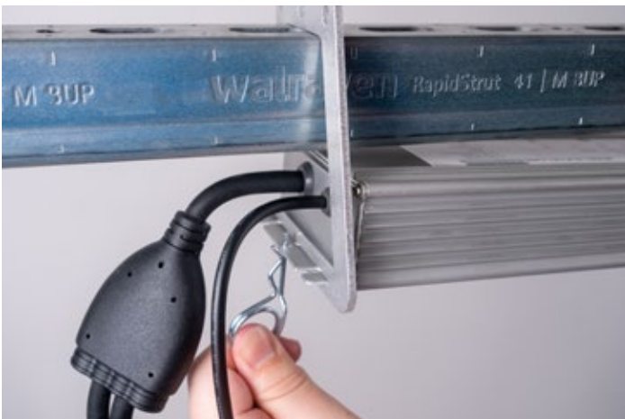
Step 5: Secure front and back end of the driver with the splints in the slot of the hanging brackets.
