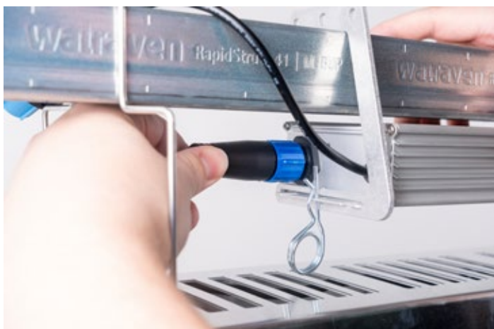
Step 8: Plug in the DC cable into the plug on the LED driver.
