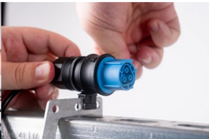
Step 10: Now you can secure the dimming signal plug.
