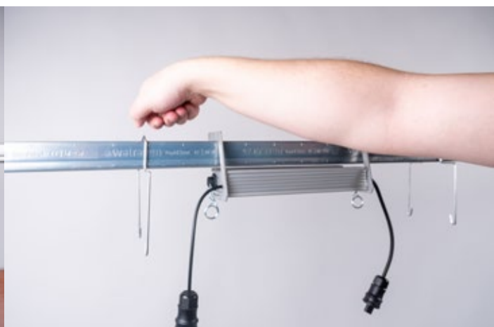
Step 6: Take the LED hanging brackets and place them left and right of the driver.
