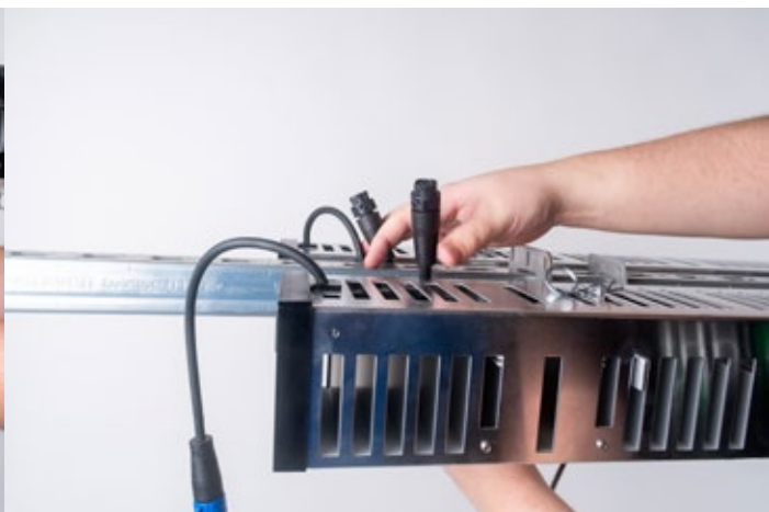
Step 11: Take the two DC cables from the driver and route them over the carrier, between the carrier and the lights.
