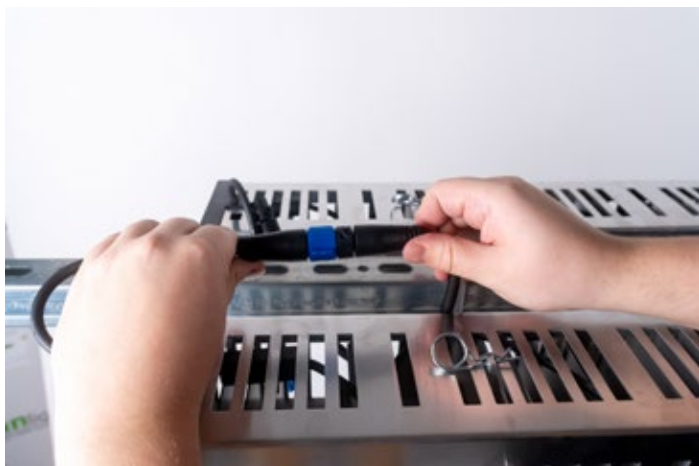
Step 11: Connect both DC cables. Make sure the plugs are orientated correctly! You will hear a 'click' sound.
